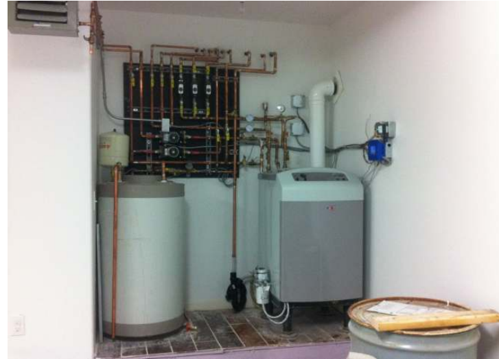
Habit for Humanity - Baseboard
