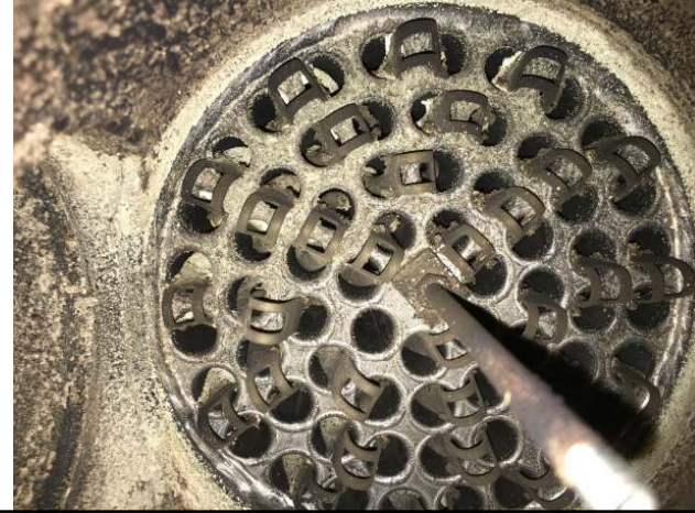
Clean System 550 Gallons Baseboard House with Tekmar 402
