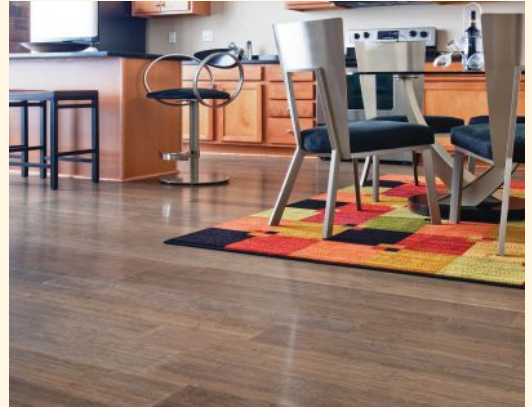
Bamboo can serve as the finishing veneer layer on an engineered wood floor, or the strips can be laminated on edge in either direction to make a solid bamboo board.
