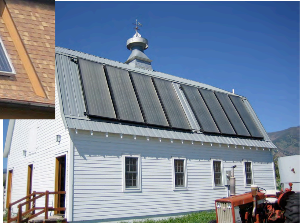
Entire collector array is sloped
