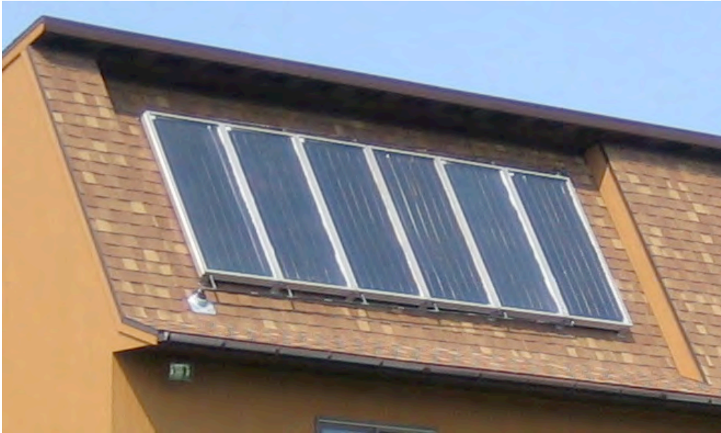
External header is sloped
