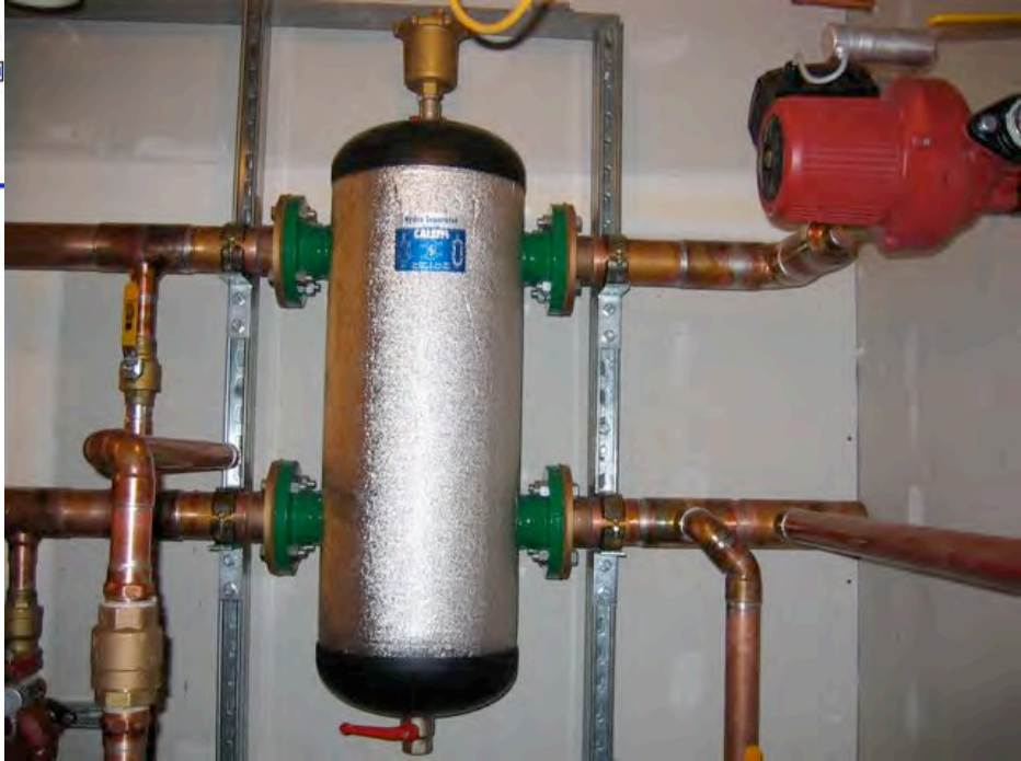
Photos courtesy of Peter Gasperini - Northeast Radiant
